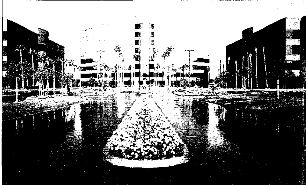
CBRE’s Class A Orange City Square property offers tenants a total office environment including retail and hotel amenities.
